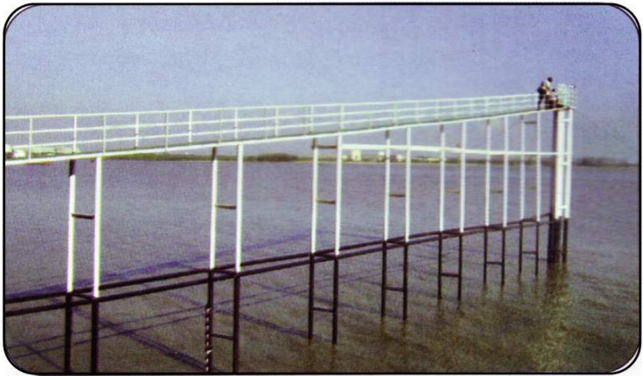
Auto Tide Gauge Station at Khal 18
