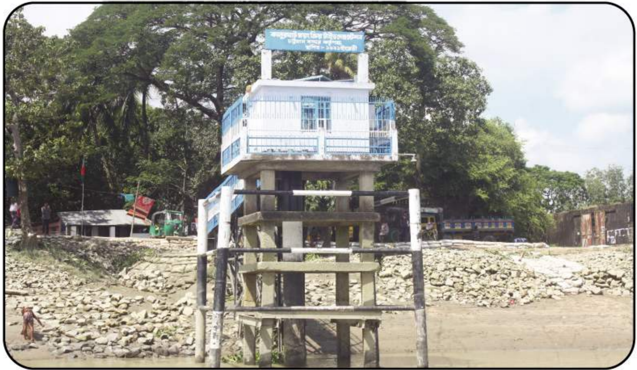
Auto Tide Gauge Station at Kalurghat
